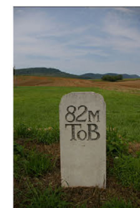
SANDBLASTED CONCRETE PEDESTAL
